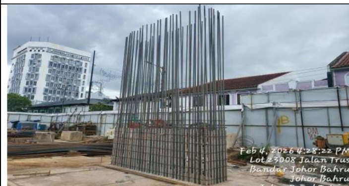
SW3 rebar installation
