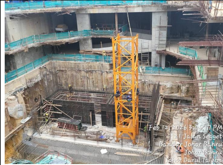
Tower crane 2nd and 3rd mast erected
