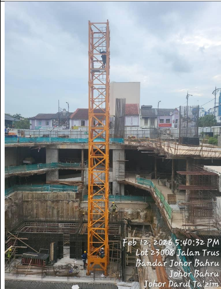
Done installing tower crane mast
