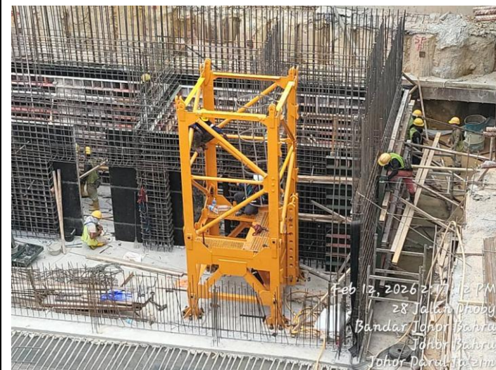
Tower crane base and 1st mast erected
